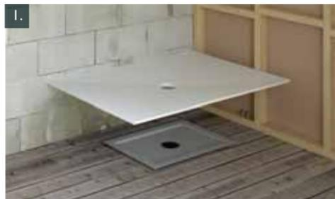
1. Place shower base in required position against wall/s and mark position of centre waste hole onto flooring. Remove base and position metal tray ensuring waste hole is centred over marked position. Mark corners of tray onto flooring. Measure and draw lines inside of marked corners, this is the area of flooring to be removed.
