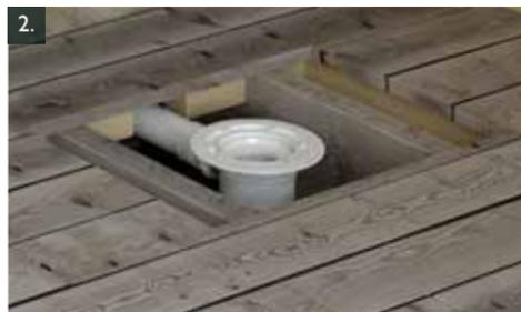
2. Using circular saw, saw depth to suit floor thickness and remove the area of floorboards. Connect waste body using 50mm/2" solvent weld waste pipe (not supplied), ensuring waste body is positioned to centre of the cut-out. Screw fix 4" x 2" (100 x 50mm) timbers (not supplied) to underside of flooring to strengthen the edges of the cut-out.
