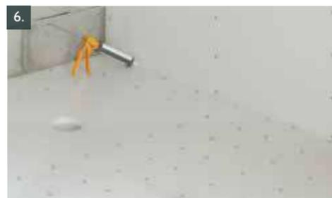
6. Apply a continuous bead of solvent weld to the edge of the shower base, as shown. Lay the first panel onto base and against the wall applying pressure to ensure the panel is fitted firmly against the base. Secure the panel in place using drywall screws at approx. 150mm centres into the stud-work, then wipe clean surplus solvent weld.
