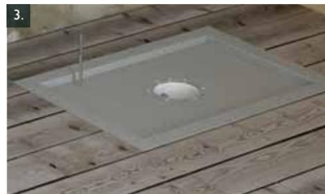
3. Mark centre lines of exposed joists onto flooring. Insert metal tray into cut-out and transfer drawn lines onto tray. Drill and countersink two holes per joist through metal tray to suit csk-head wood screws (not supplied). Screw metal tray into position.
