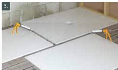
5. Using KUDOS Solvent Weld, apply a continuous bead to the edge of the shower base, as shown. Lay the first aqua4ma panel up to the edge of the base applying pressure to ensure the panel is fitted firmly against the base edge. Secure the panel in place using drywall screws at 150mm centres, then wipe clean surplus solvent weld. Joints should be staggered, as shown to help strengthen the overall assembly.
