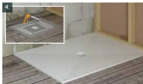
4. Apply beads of KUDOS Grabber Adhesive to base of metal tray and the 4 outer flanges as shown. Carefully position shower base into position and stand on it to ensure it is fully bedded down onto tray and floor. Secure in place by using drywall screws (not supplied) around the perimeter at 150mm centres ensuring these avoid the metal tray underneath.
